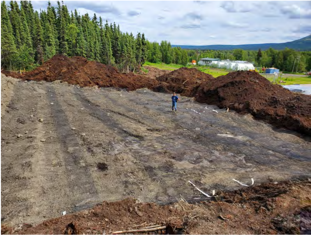
Photograph 3: Photograph of Geogrid laid over leveling course.
