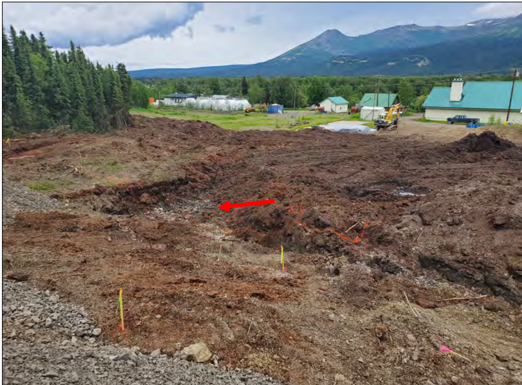
Photograph 1: Proposed pad footprint (orange paint) looking south, northwest corner in foreground with existing excavation partially within footprint (red arrow).
