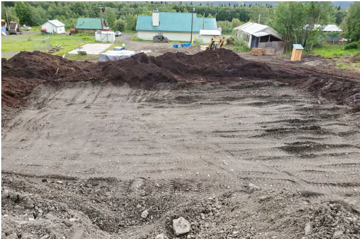
Photograph 5: Fill pad after compaction of first lift.
