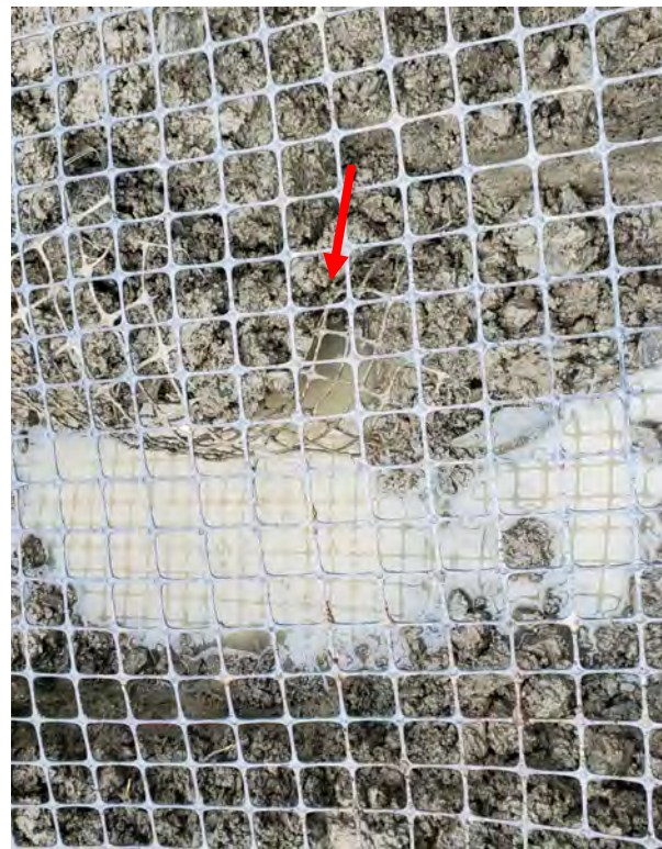
Photograph 6: Photograph of exposed, potentially damaged Geogrid (arrow), with repair patch overlaid.
