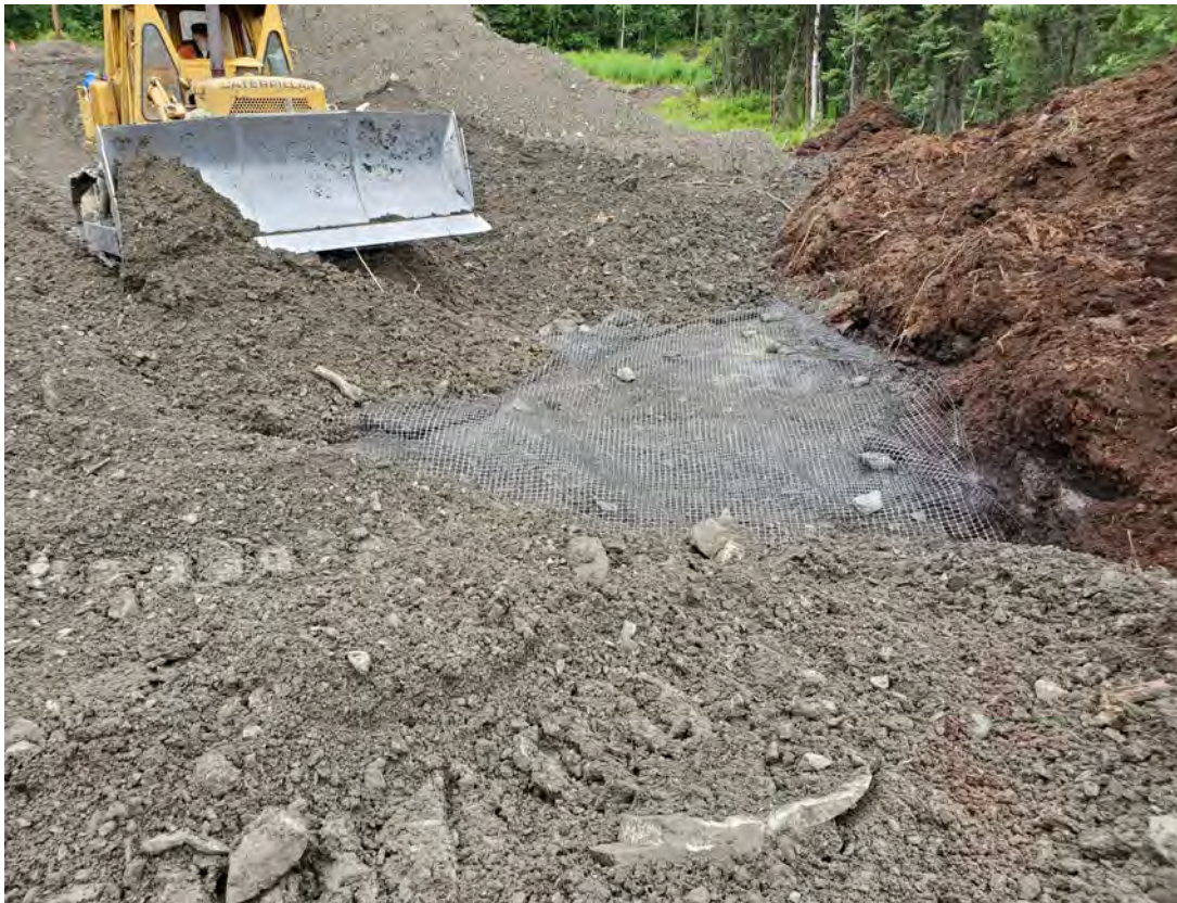
Photograph 4: Photograph of fill placement over Geogrid (first lift).
