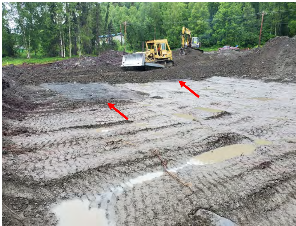
Photograph 8: Photograph of fill placement over Geogrid repair patches. View is looking west, location of repairs indicated with red arrows.
