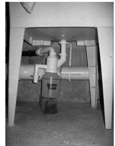
Misaligned installation
