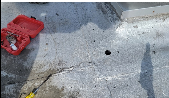
Photo 1. Sample AS-02 – Central Roof; Roofing Materials.
