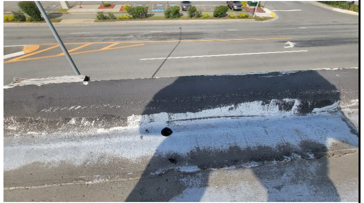
Photo 4. Sample AS-05 – Northwest Roof; Roofing Materials.
