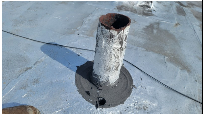
Photo 2. Sample AS-03 – Central Roof; Roofing Materials.
