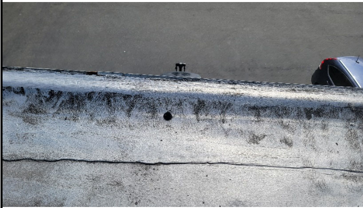
Photo 3. Sample AS-04 – Southeast Roof; Roofing Materials.
