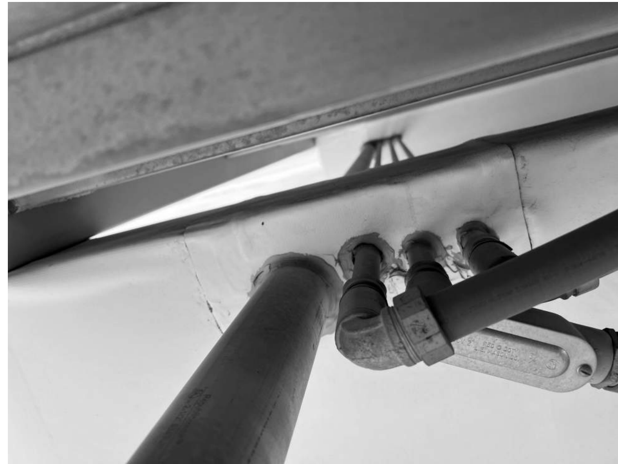
ROOF E - AHU CURB PENETRATIONS
