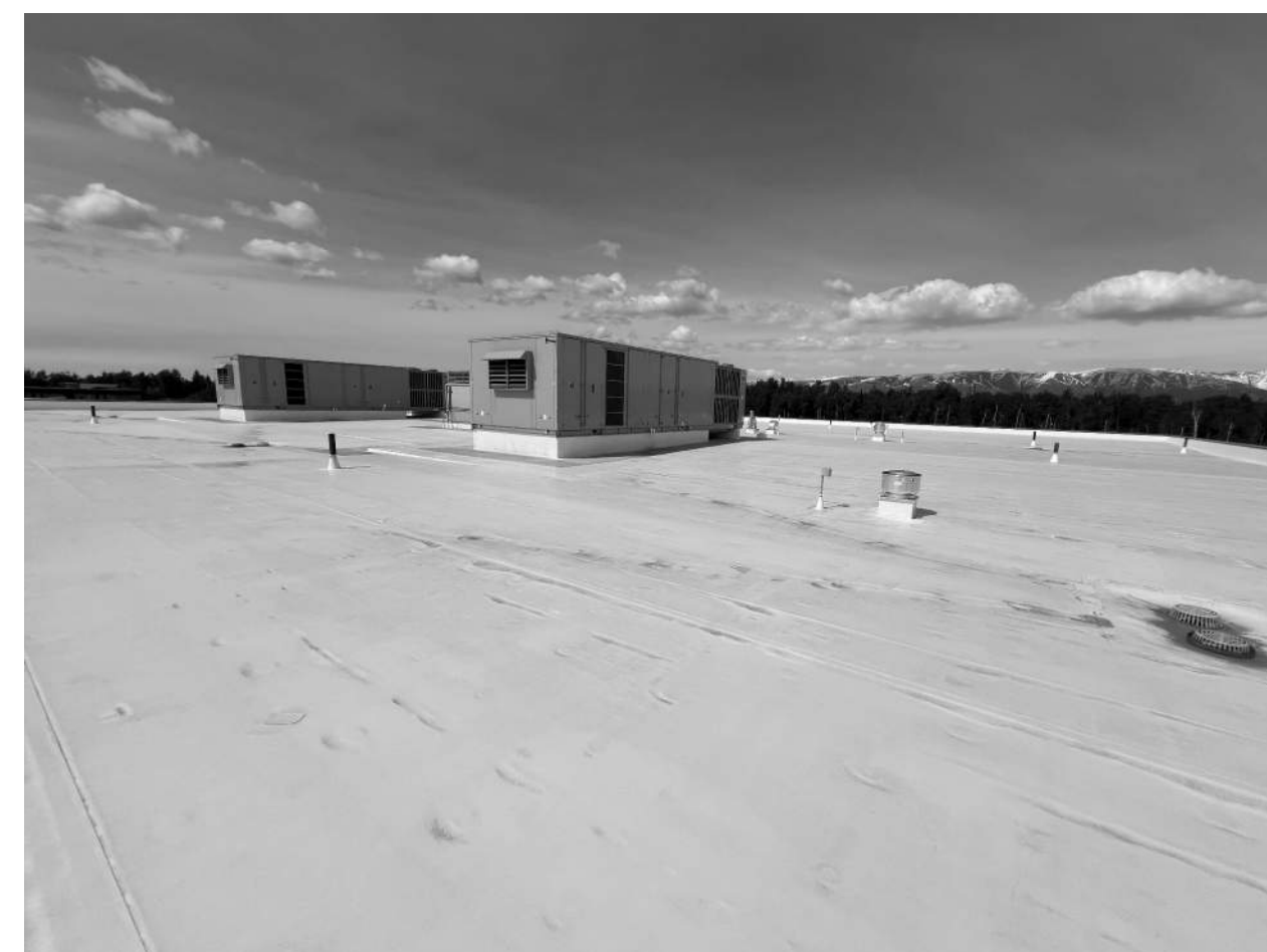
ROOF E - FROM SE CORNER
