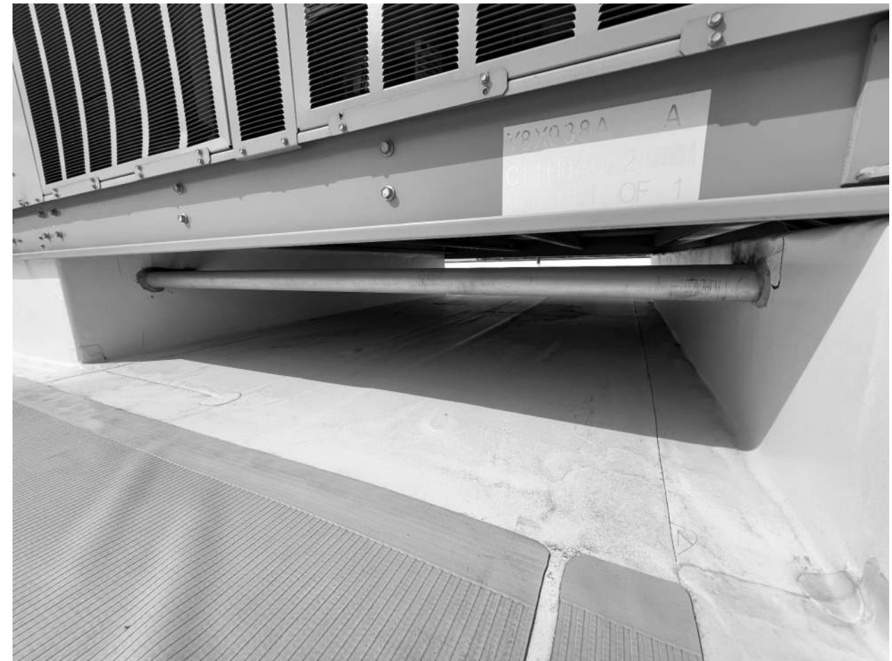
ROOF E - AHU CURB PENETRATIONS
