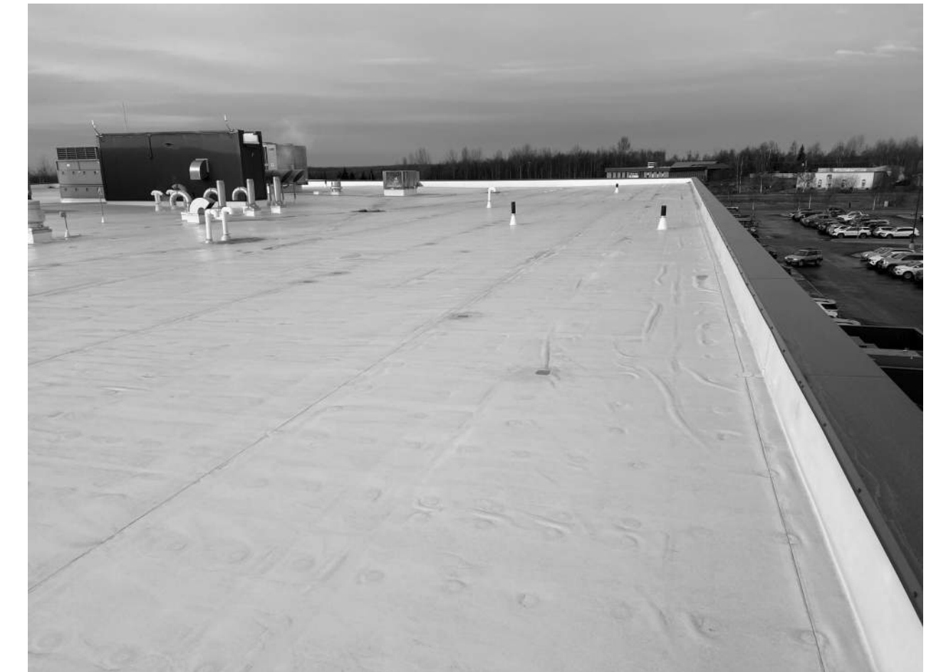
ROOF E - FROM NE CORNER
