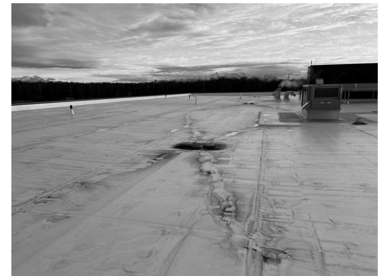
ROOF E - FROM NW CORNER
