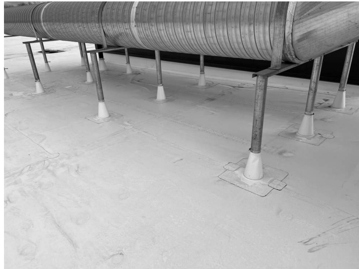
ROOF E - DUCT SUPPORTS
