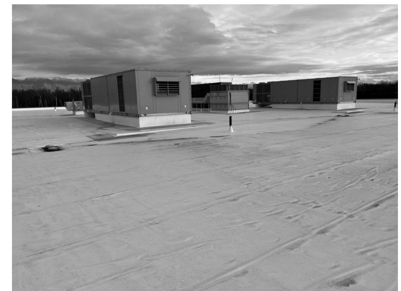
ROOF E - FROM SW CORNER
