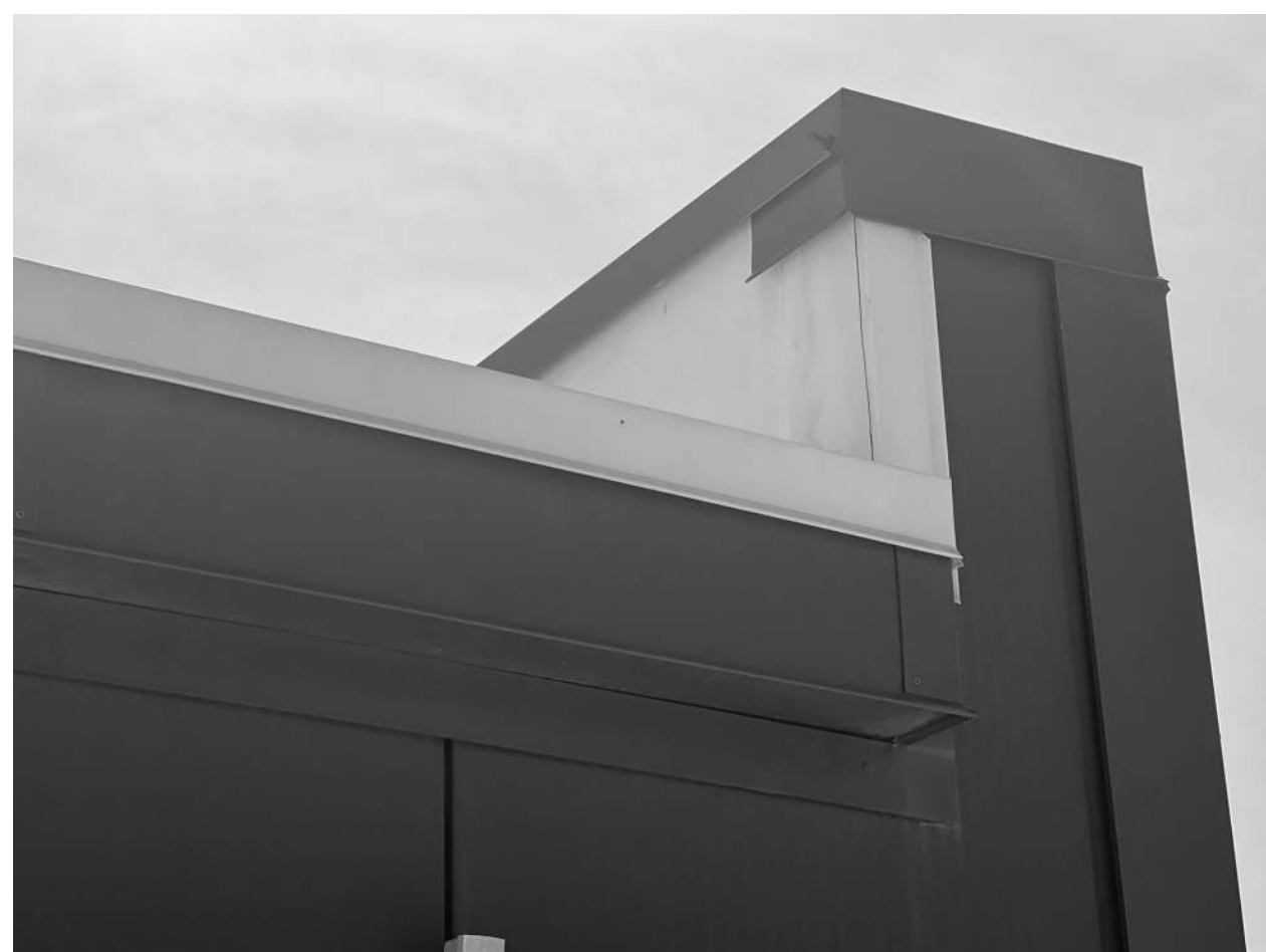
ROOF E - STAIR ROOF
