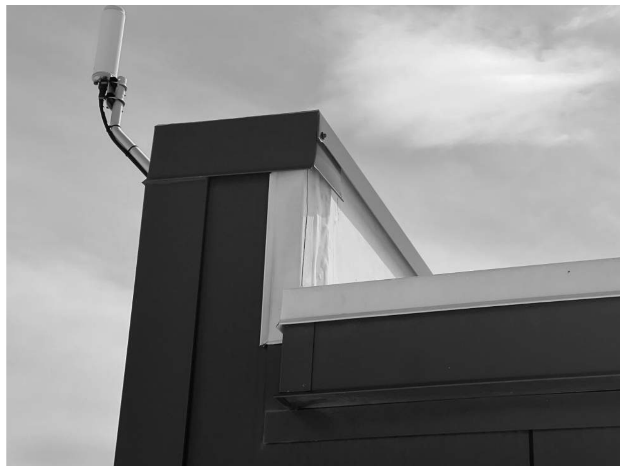
ROOF E - STAIR ROOF
