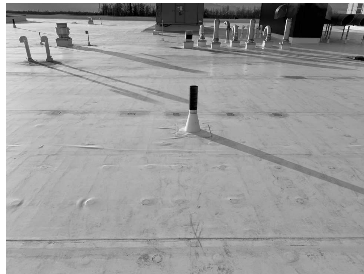
ROOF E - LOOKING SOUTH
