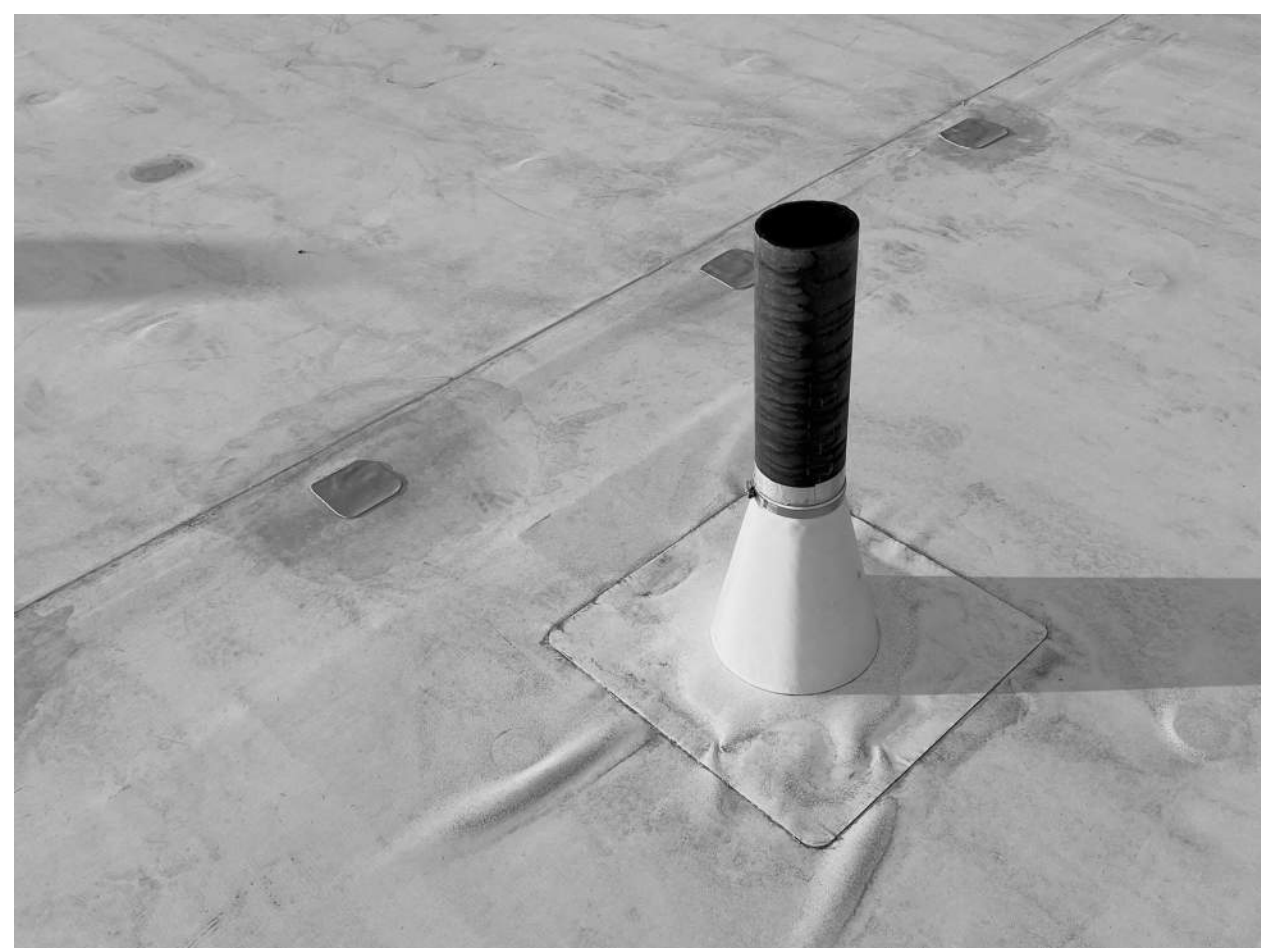
ROOF E - TYPICAL VTR
