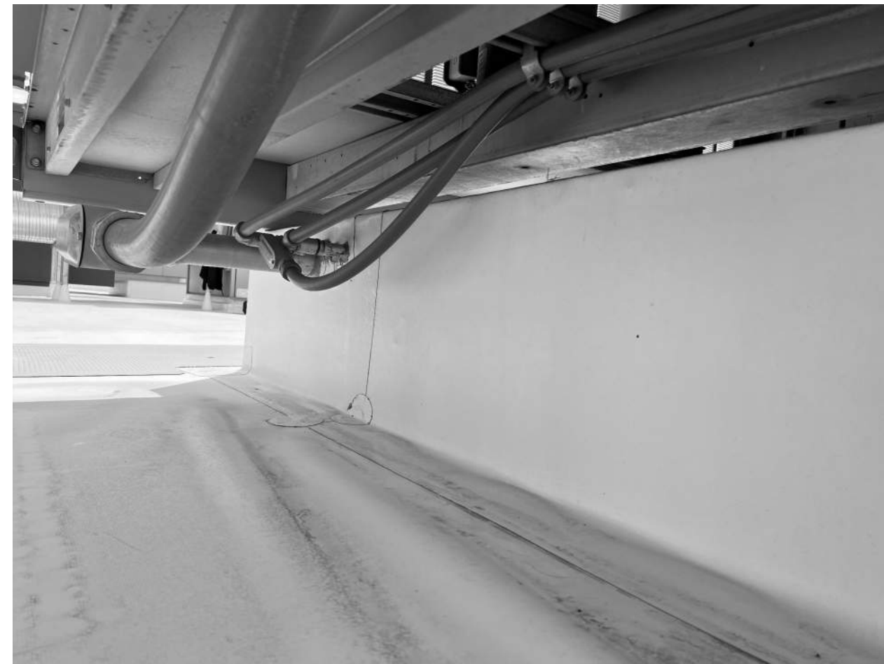
ROOF E - AHU CURB PENETRATIONS
