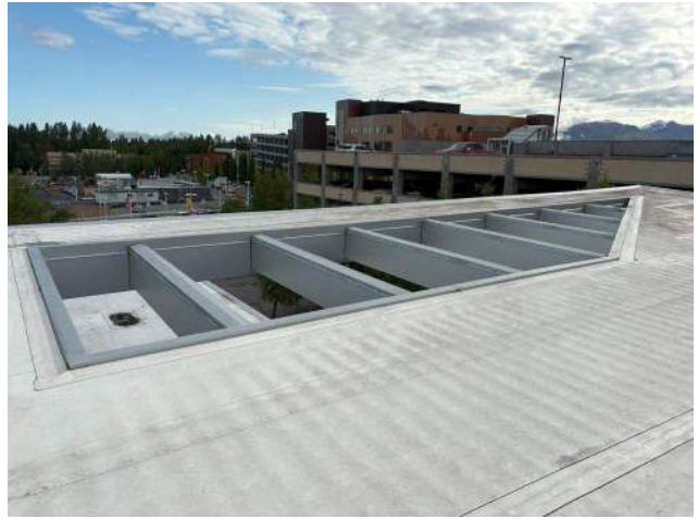
PCC 3 Roof – openings at northeast corner
