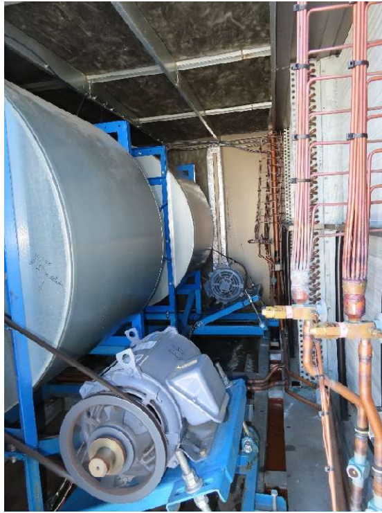
PCC3, RTU-2 VFD drives shown at left, 1 for each of 2 supply fan motors, shown at right and 1 for the return fan motor (not shown)
