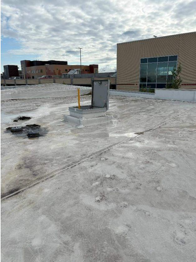
PCC 3 Roof – access hatch
