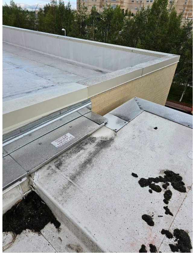
PCC 1 Roof – seismic joint at east addition
