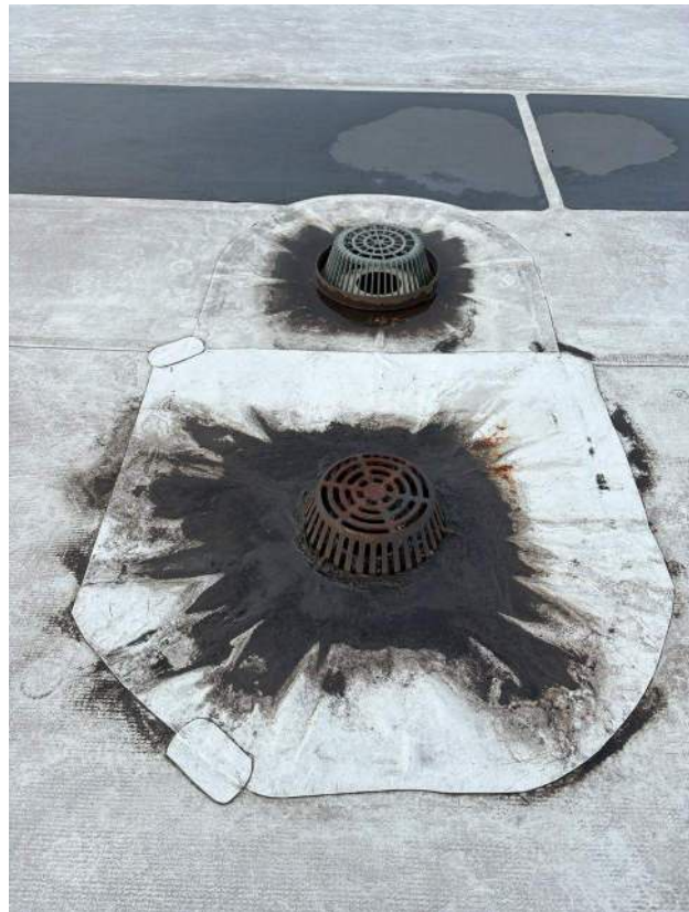
PCC 2 Roof – typical roof drain
