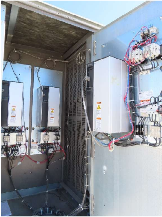
PCC3, RTU-2 VFD drives shown at left, 1 for each of 2 supply fan motors, shown at right and 1 for the return fan motor (not shown)
