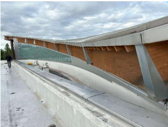
Atrium – from PCC1, looking southwest
