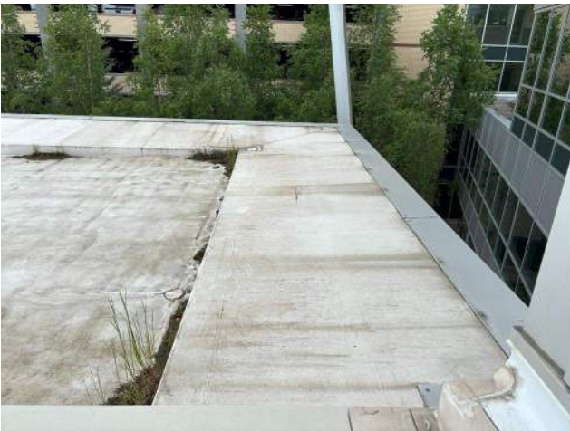
PCC 1 Roof - east addition
