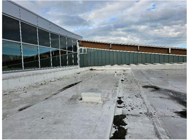
PCC 1 Roof – southwest corner
