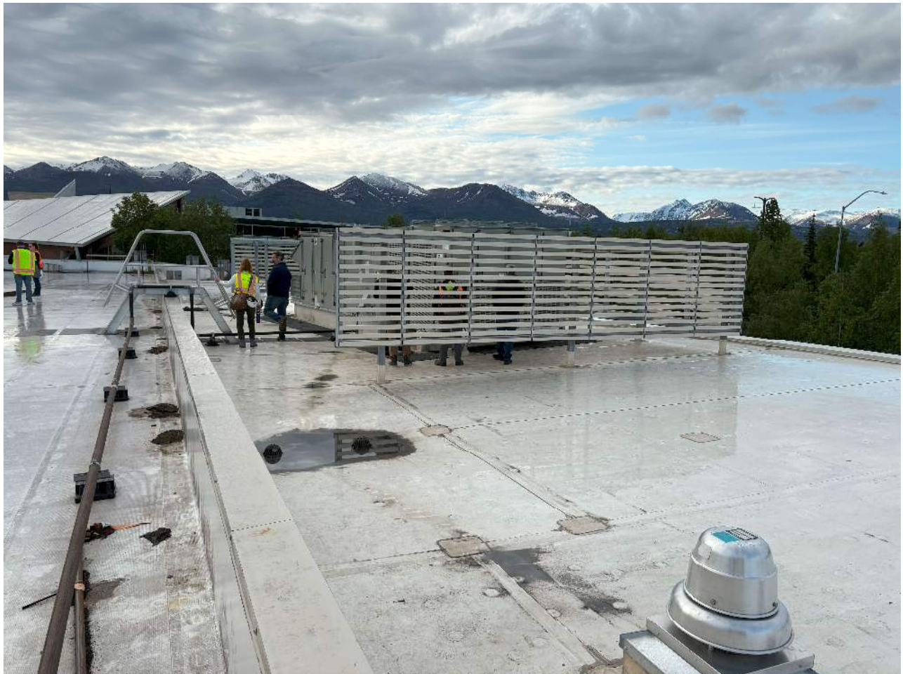
PCC 2 Roof – 2022 addition and RTU-2.4 surrounded by equipment screen
