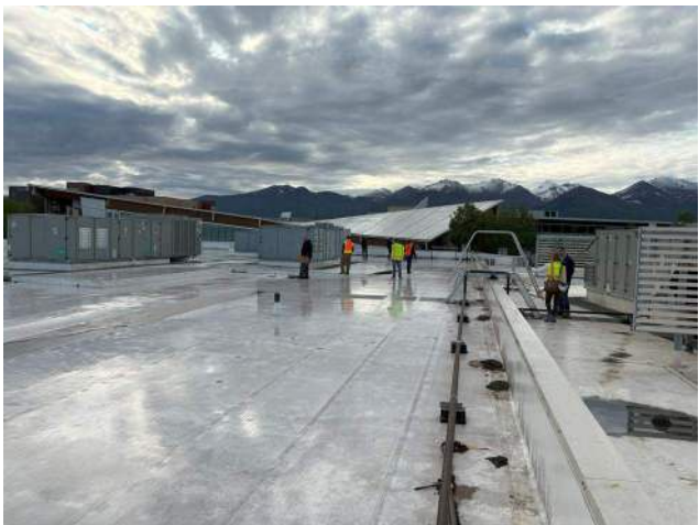
PCC 2 Roof – south side, looking east
