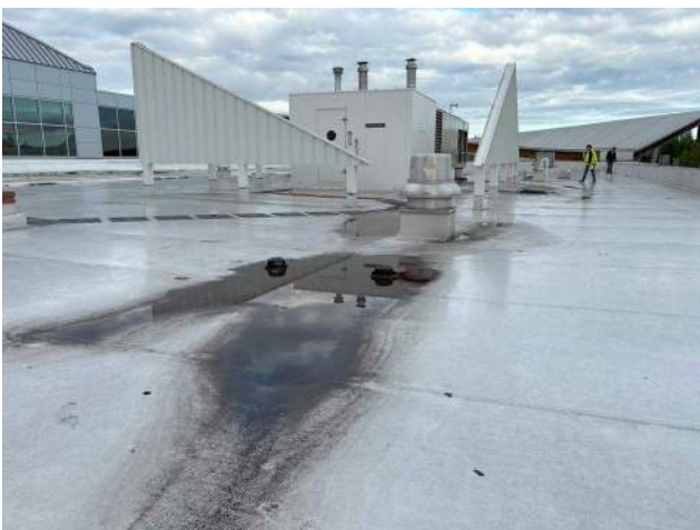
PCC 1 Roof – at northeast corner, looking west
