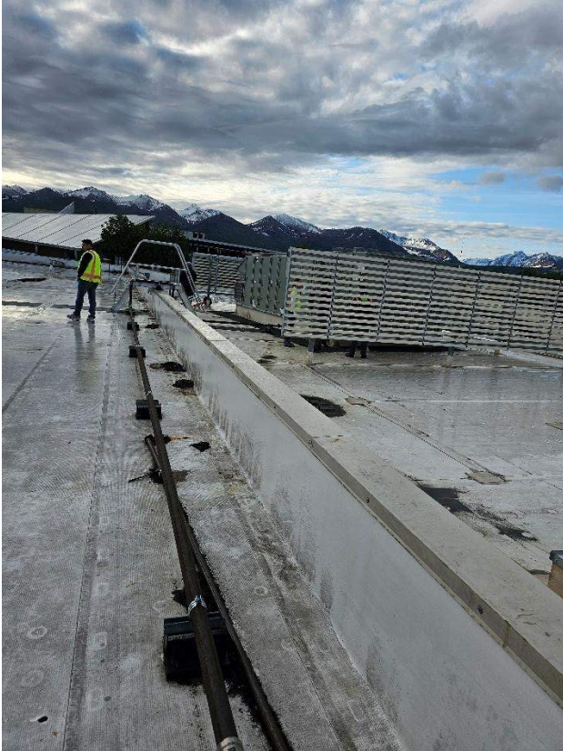
PCC 2 Roof – parapet wall at new addition
