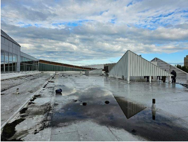
PCC 1 Roof – at southeast corner, looking west
