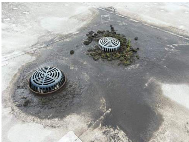
PCC 3 Roof – typical roof drains
