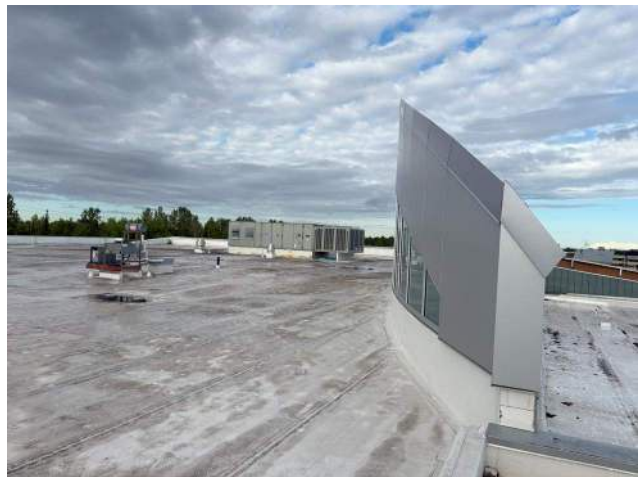
PCC 3 Roof – view from northeast subsection
