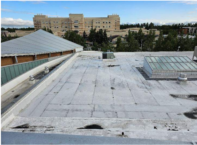
PCC 1 Roof – west side
