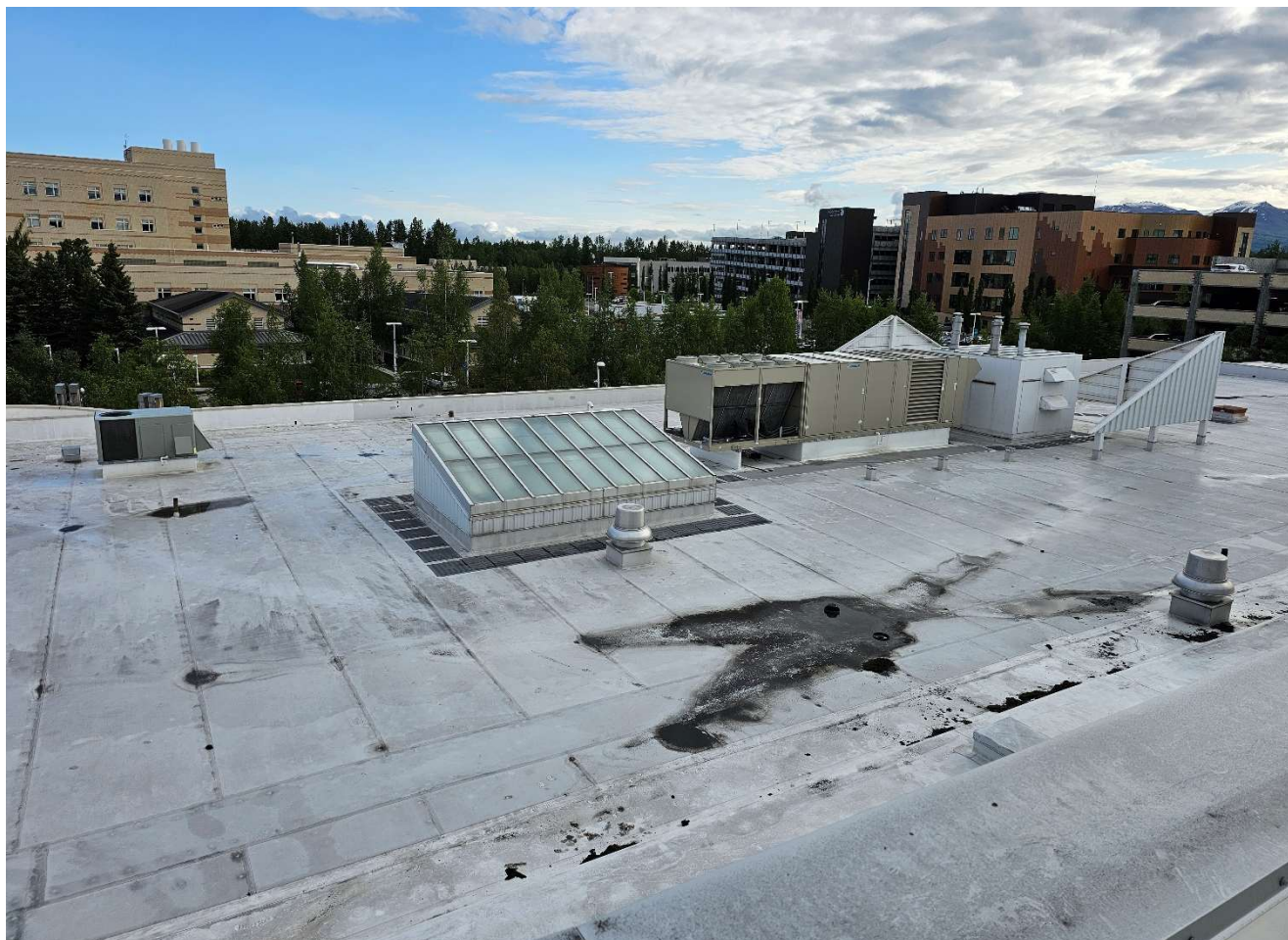
PCC 1 Roof – facing northeast
