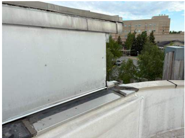
PCC 1 Roof – seismic joint at Atrium
