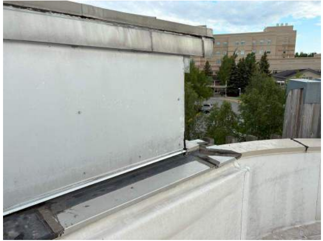
Atrium – northeast corner edge condition
