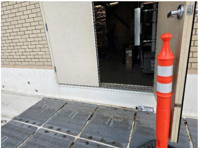
PCC 2 Roof – Boiler room entrance door
