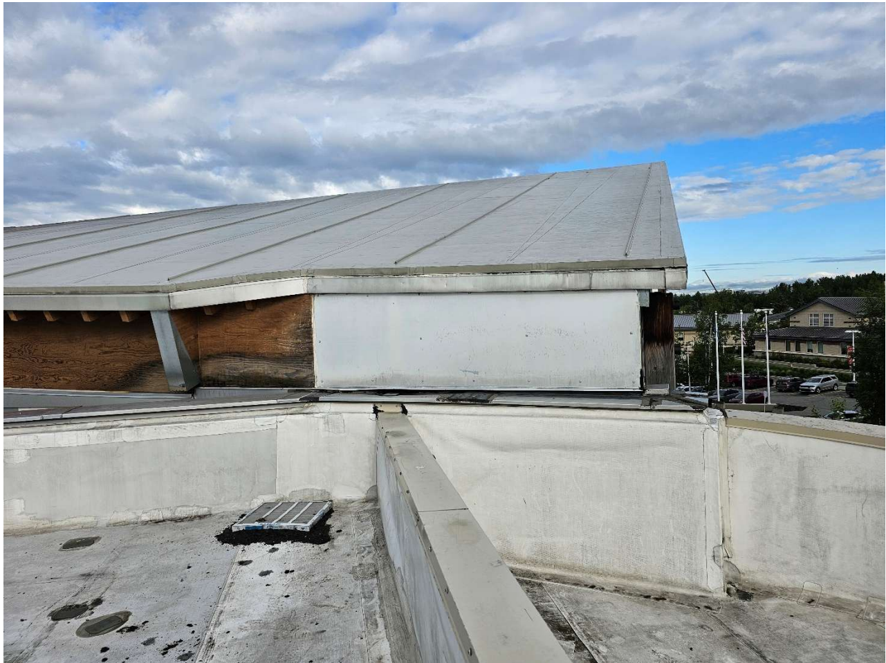
PCC 1 Roof – northwest corner – Atrium roof snow shed zone
