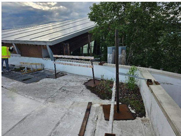
PCC 2 Roof – southeast corner of main roof
