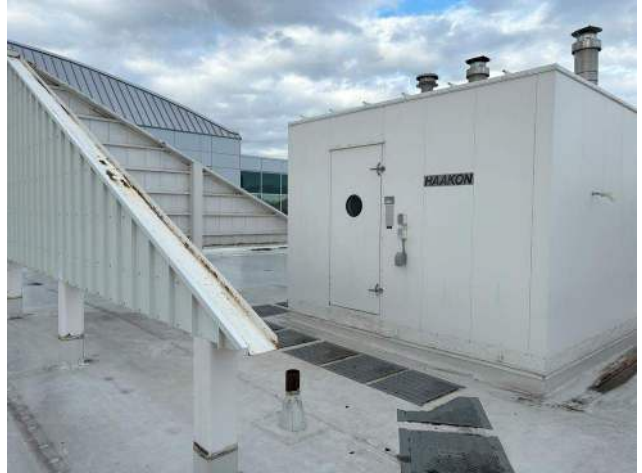
PCC 1 Roof – Boiler room module
