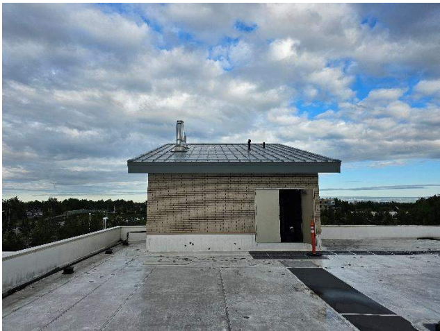
PCC 2 Roof – southwest corner, boiler room
