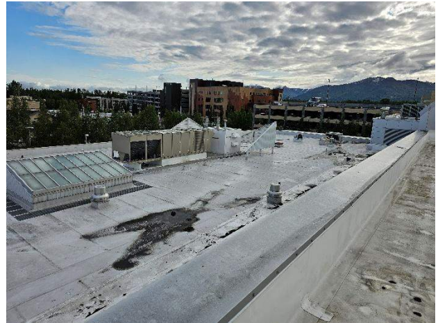
PCC 1 Roof – looking northeast
