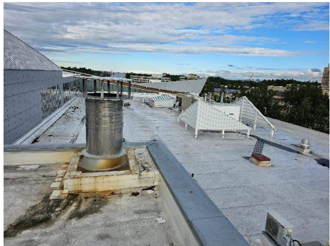
PCC 3 Roof – northeast subsection, exhaust stack
