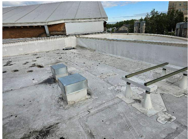
PCC 1 Roof – northwest corner
