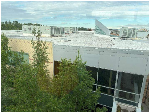
PCC 3 Roof – view looking north from parking garage
