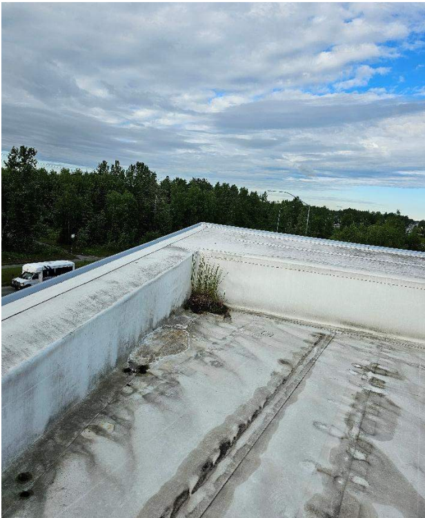
PCC 3 Roof – southwest corner
