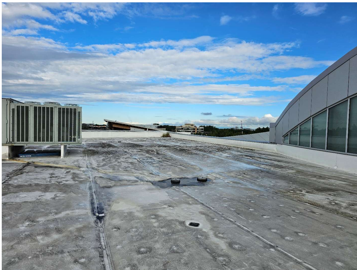
PCC 3 Roof – facing west
