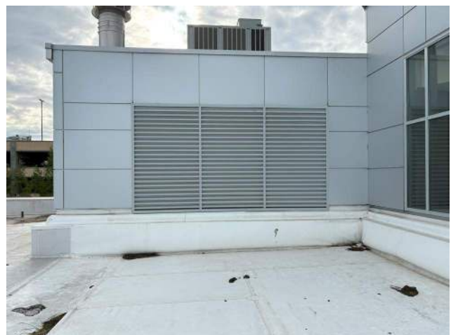
PCC 1 Roof – southeast corner
