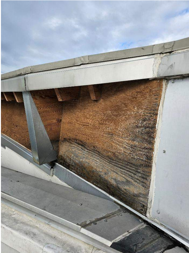
Atrium – northeast corner at PCC1 seismic joint
