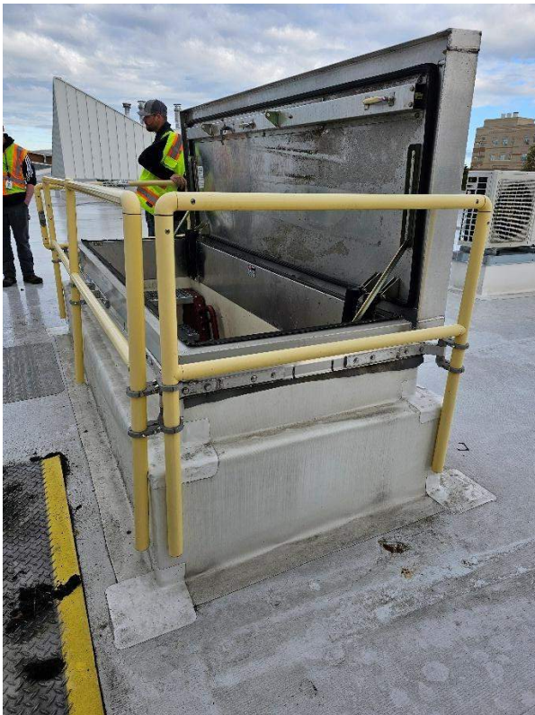
PCC 1 Roof – Access hatch
