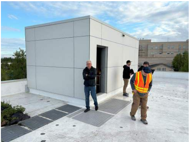
PCC2 Roof – northwest corner, stair access
