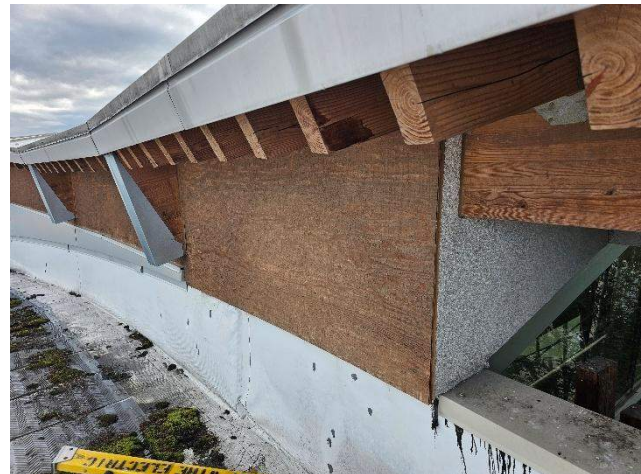
Atrium – southwest corner eave condition
