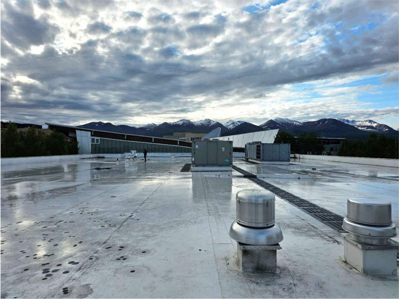
PCC 2 Roof – facing east
