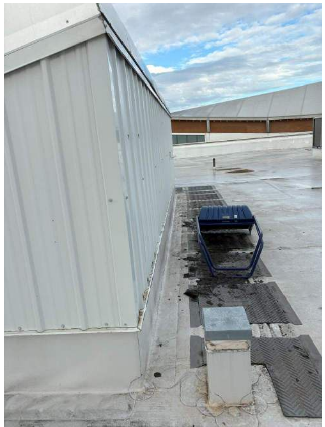
PCC 1 Roof – north (peak) side of skylight
