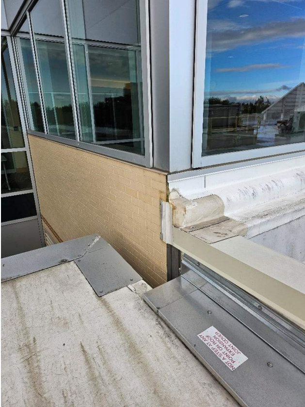
PCC 1 Roof – seismic joint at east addition
