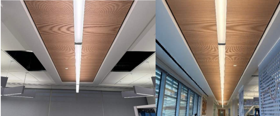
Figure 5: Open Office areas with wood-look perforated ceiling panels
